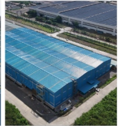
Completion of HR Coil Warehouse with 70,000 tons capacity on a 16,000 m² area to transform logistics and supply chain efficiency.
